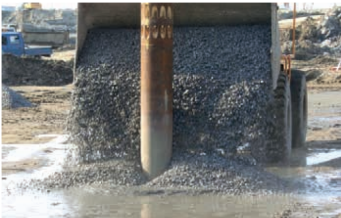
Backfilling at ground surface wet “Top Feed”
