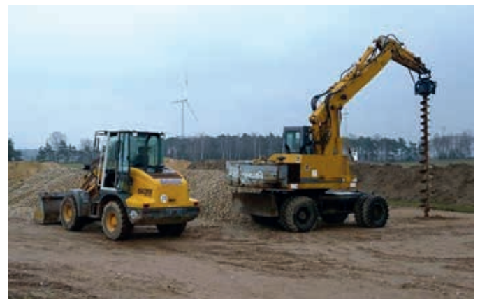
Pre-boring operation with auger
