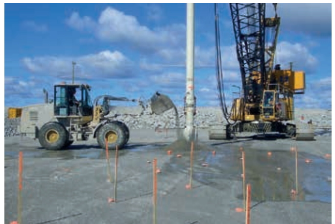
Placement of backfill material by a wheeled loader
