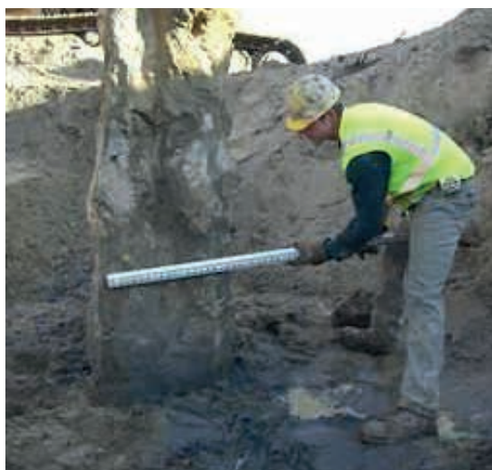
Excavated VCC column
