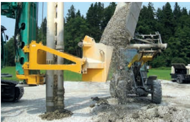
Backfilling via the material transfer unit
