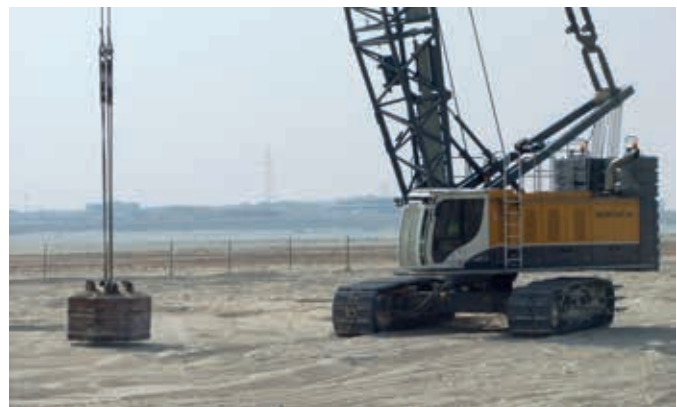
Drop height 25 meter, pounder weight 20 tonnes
