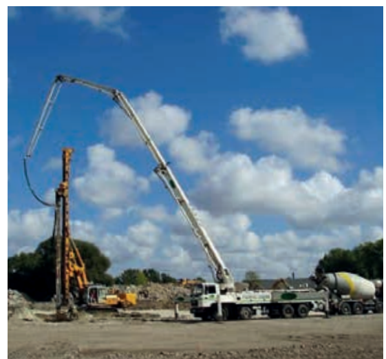
Concrete placement for VCC column
